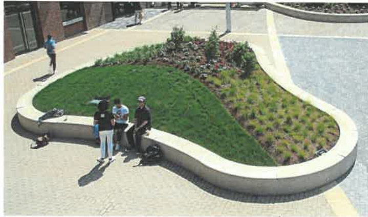
Raised Concrete Planter/Seatwall
