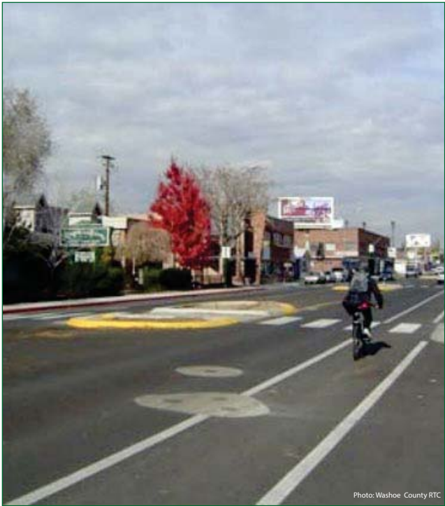
Wells Avenue after the completion of the Road Diet.
