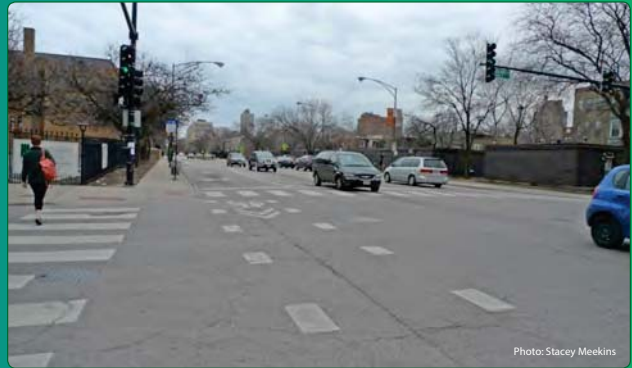
Bus stop and shared lane at intersection, through intersection markings
