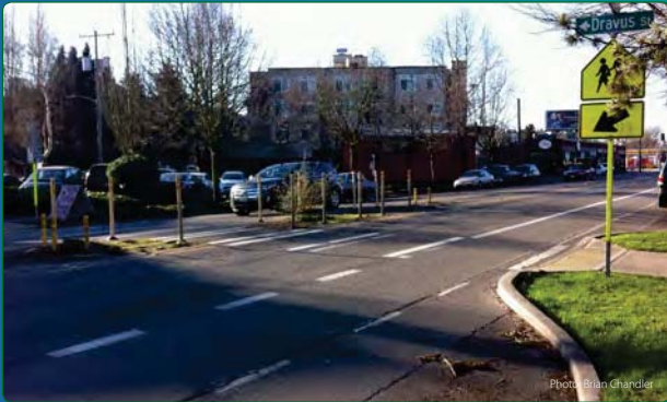
To improve pedestrian safety, the Road Diet project incorporated crosswalks with curb bulb-outs and pedestrian refuge islands
