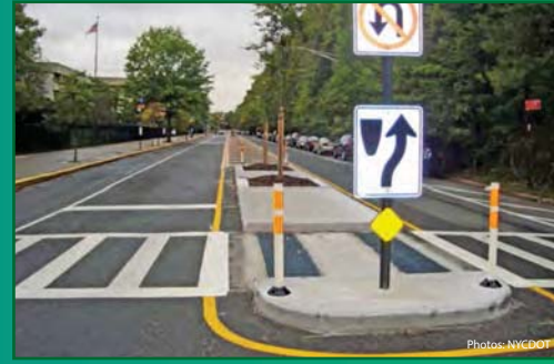
A pedestrian refuge island improves safety for pedestrians near Tottenville High School.
