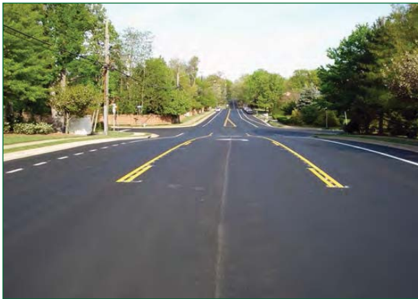
Oak Street after installation of Road Diet markings
