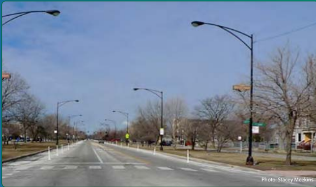
3-lane cross-section with bollard-separated bicycle lanes
