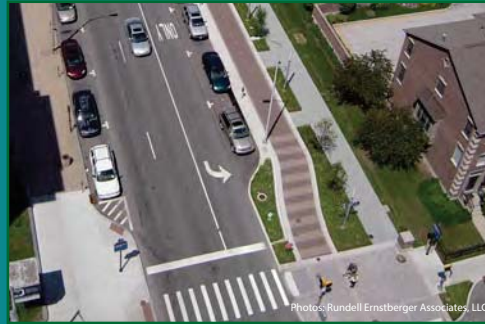
Pedestrian travel is separated from bicycle travel on this segment of ICT.
