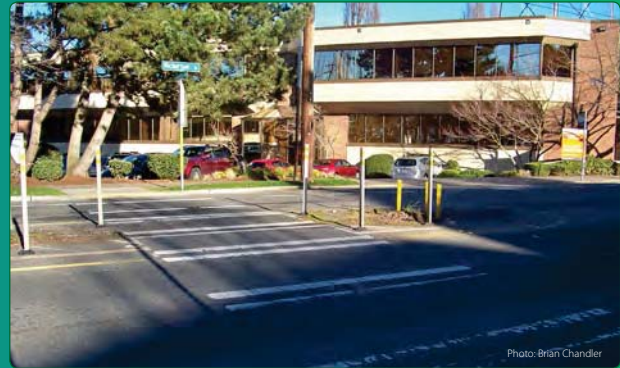
To improve pedestrian safety, the Road Diet project incorporated crosswalks with curb bulb-outs and pedestrian refuge islands
