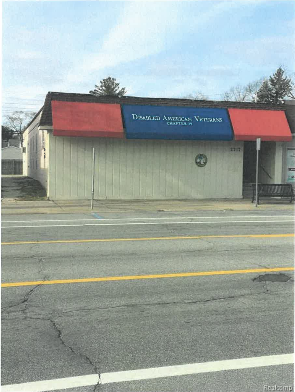
PRIOR FAÇADE CONDITION OF 2717 COOLIDGE
